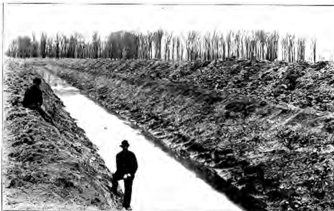
DRAIN EIGHT FEET BOTTOM WIDTH, EIGHT AND ONE HALF FEET DEEP, CONSTRUCTED BY DREDGE SHOWN IN PLATE V. IN 1917, AT COST OF \$2.25 PER ROD (ABOUT 8 00/100 PER CUBIC YARD) TO REPLACE SHALLOW TEAM AND SCRAPER DRAIN CONSTRUCTED IN 1914 AT A COST OF \$1.00 PER ROD.
