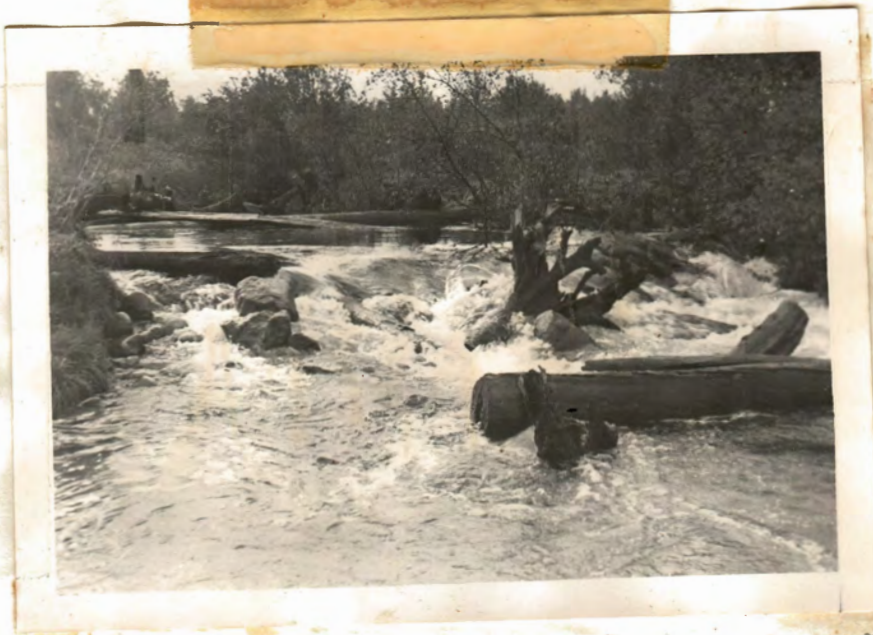
United States Park Service work in Pigeon River. A high-face dam of this type is likely to silt in and be damaged by ice action.
