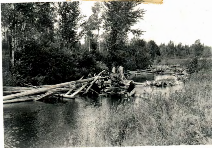
United States Park Service work in Pigeon River, "Hay field" section. Such installations cannot operate efficiently, or fulfill definite purposes, because of their lack of coordination in design, and lack of adequate moorings, which allows them to change position.
