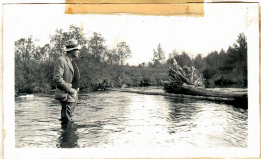
United States Park Service work in the Pigeon River. Where the water is seen to be knee deep it was formerly hip deep, due to an efficient wing deflector. The hole produced by it is filled in since the deflector was removed by the U.S.P.S. The log jam seen across the stream will cause fishermen much annoyance since it interferes with fly fishing.
