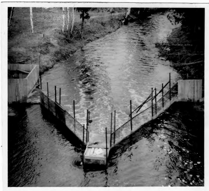
Figure 6. Carp Creek weir, May 5, 1947. Note damming action of weir screen prior to cleaning. This screen had been cleaned six hours earlier.
