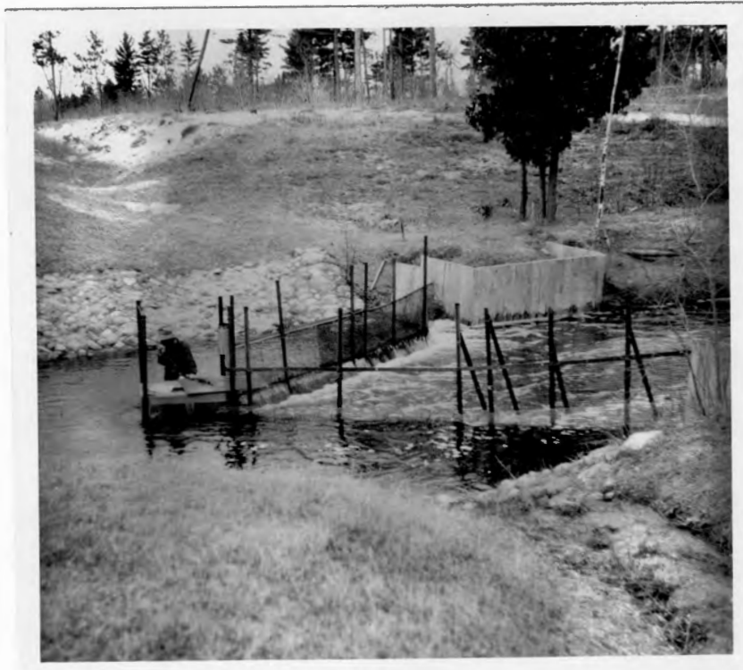
Figure 6. Carp Creek weir, May 5, 1947. Note damming action of weir screen prior to cleaning. This screen had been cleaned six hours earlier.
