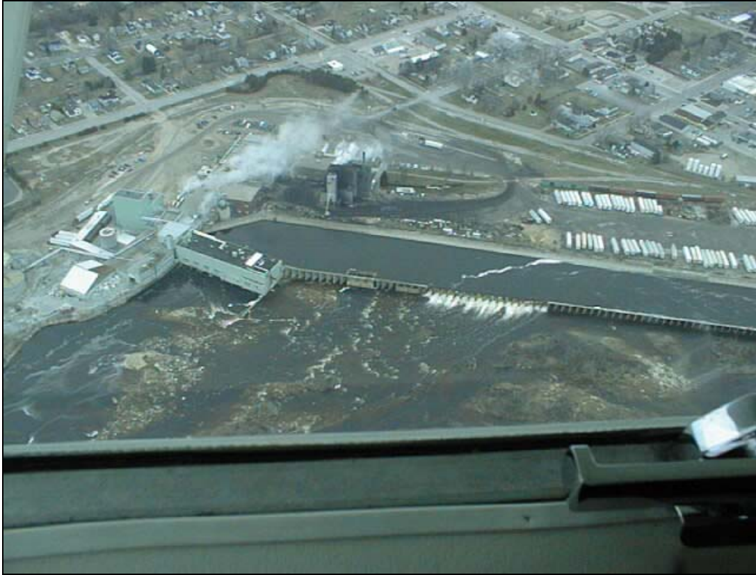
Downstream View of MPI Dam
