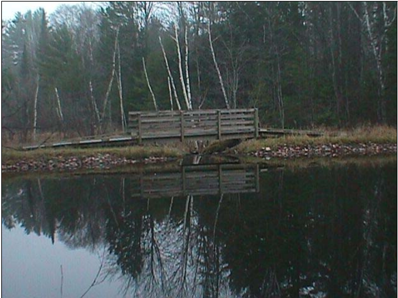
Council Lake Dam
