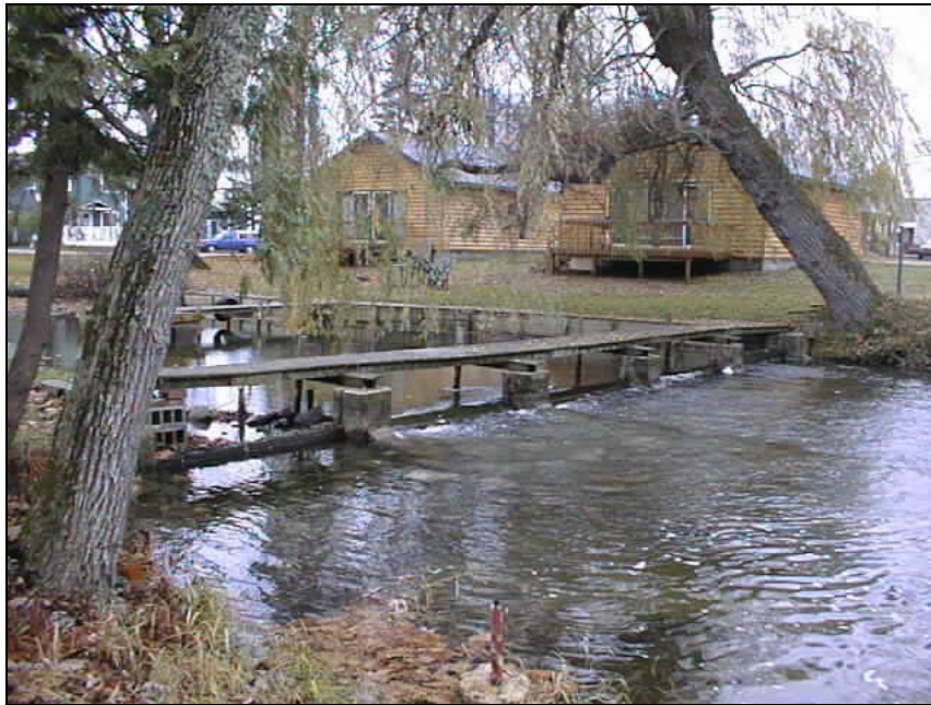
Portage Creek Dam (South Manistique Lake) at low flow with all stop boards removed.
