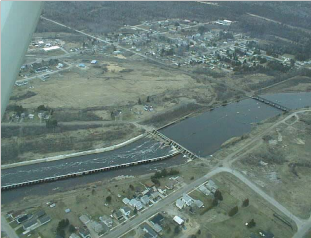
Upstream View of MPI Dam
