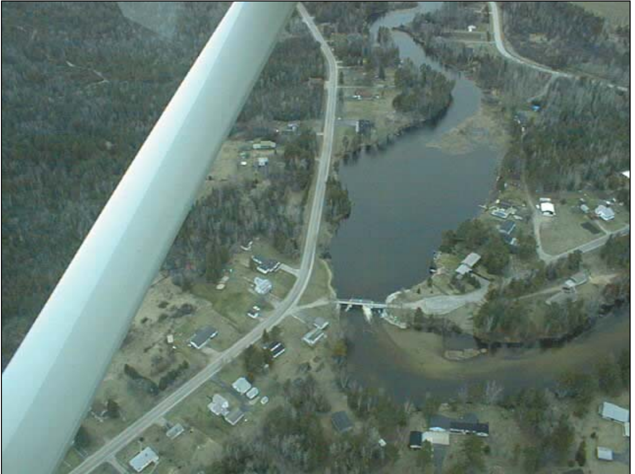
Indian Lake Dam
