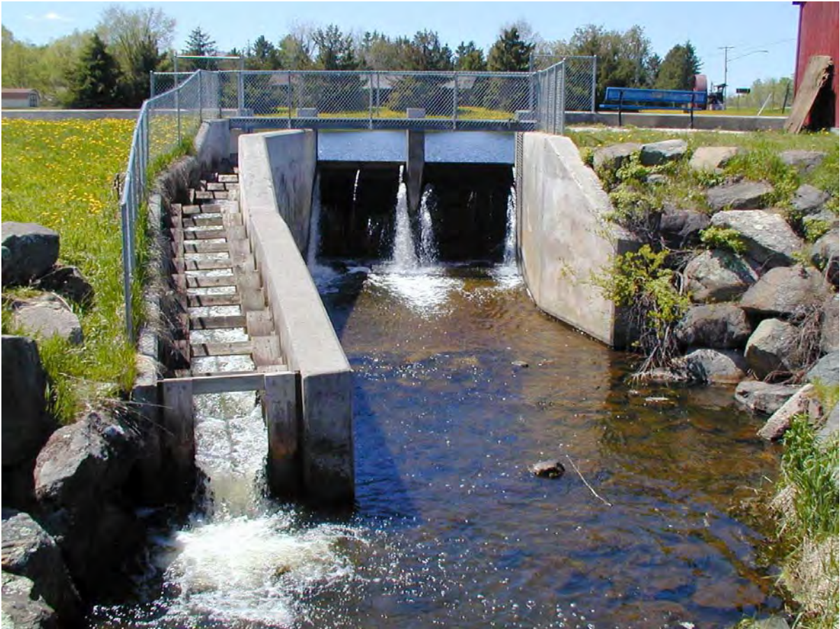
Photo 2.—Trout Creek Dam and fish ladder.
