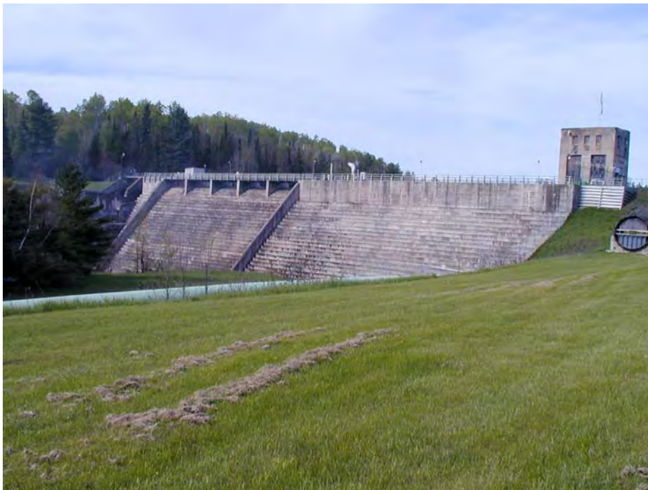
Photo 4.–Victoria Dam, West Branch Ontonagon River.
