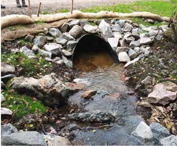
Good (large rip rap covers entire flood prone area)
