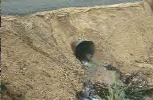
Severe embankment erosion, mass wasting
