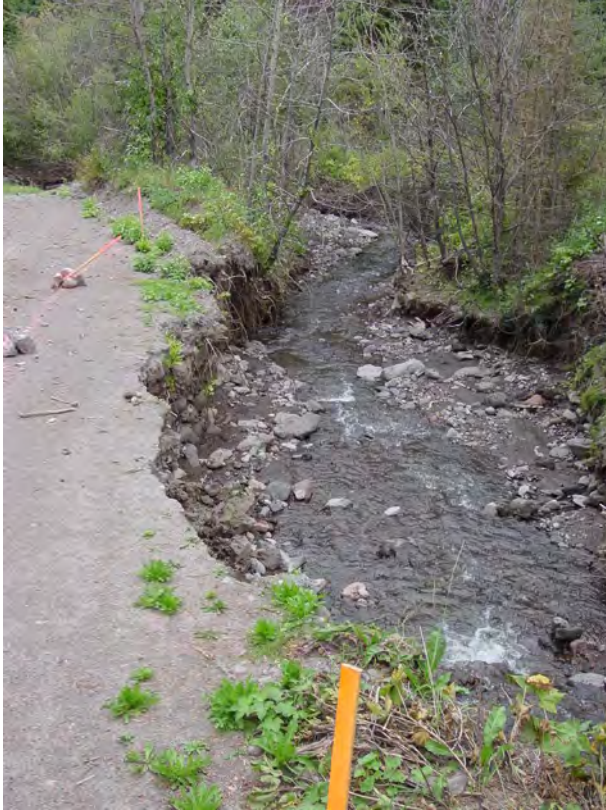
Severe embankment erosion, mass wasting
