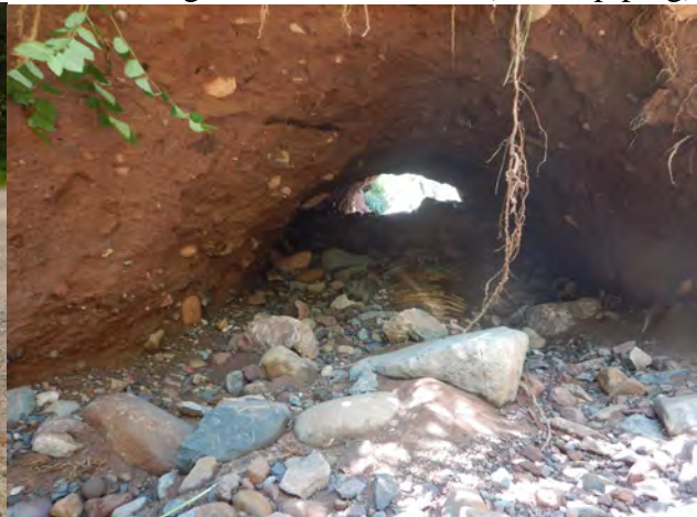
Undermining/subsurface erosion (severe piping)
