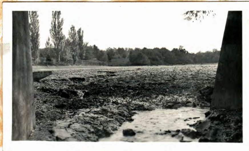
Fig. 6. View of pond bottom from dam
