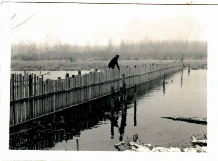
Looking downstream at the main arm of the Muskegon River weir showing the braces above the weir. This picture was taken by Dr. J. W. Leonard just after the weir was completed and before the traps had been moved out in river from their original position partially buried in either bank.
