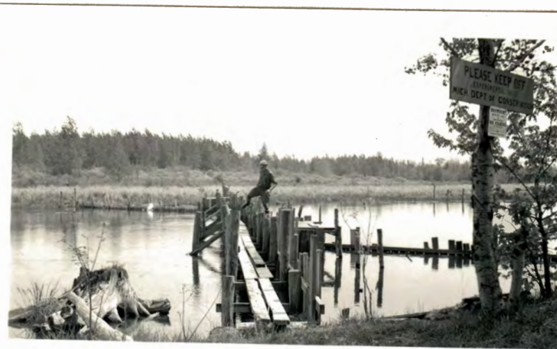
Side view of the Muskegon River weir showing catwalk, the main arm of the weir with braces, and the short wings leading from the bank to each trap. Mr. Harold Bowditch, facing downstream, is stepping from the downstream trap to the catwalk.
