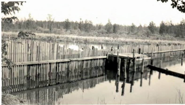
Front view (looking downstream) of the Muskegon River weir, showing the construction of the downstream trap, the main arm of the weir, and the small wing leading directly from the south bank to the trap.
