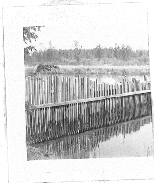
1. Downstream view of the Muskegon River Weir
