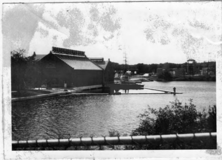
Figure 25.--Boom above power plant at Uroton Dam, Muskegon River
