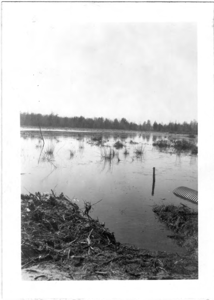
Figure 7. Photograph taken April 15, 1952 looking westward at Section A from the south end of fill No. 1. Downstream end of Culvert No. 1. in the right foreground with water level gage No. 3 just beyond its mouth. U. S. G. S. gage level 2.07 feet (1274.07 feet m.s.l.). Heavy spawning action was going on in this section at the time.
