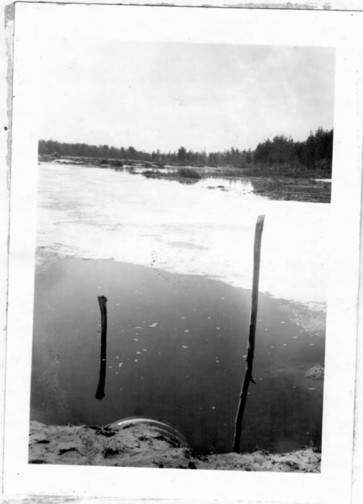
Figure 5. Photograph taken April 15, 1952 looking westward at Section B from the south end of fill No. 2. (same location as Figure 4, but one week later). Downstream end of Culvert No. 2 in foreground. Nail in left side of stake in left foreground indicates the stipulated height of the top of the culvert, or 1274.5 feet m.s.l. U. S. G. S. gage reading 2.07 feet (1274.07 feet m.s.l.). Heavy spawning action was going on at this time in the open water in the background, beyond the ice.
