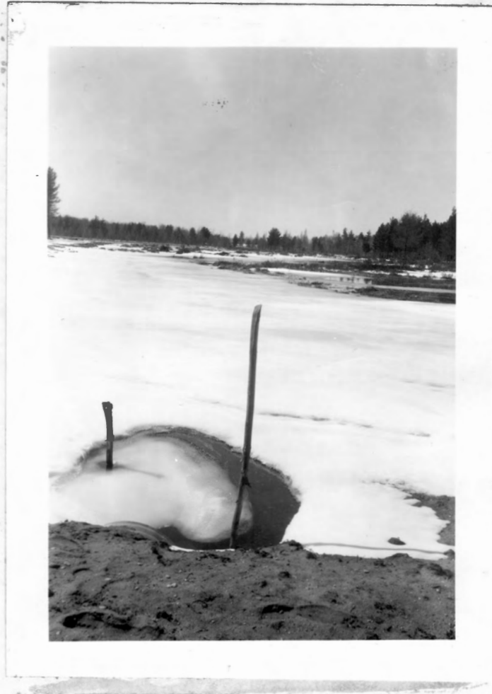
Figure 4. Photograph taken April 8, 1952 looking WF eastward at Section B from the south end of fill No. 2. Downstream end of Culvert No. 2 in foreground. U. S. G. S. gage reading 1.90 feet (1273.90 feet m.s.l.).
