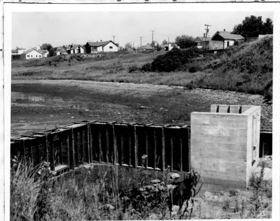
Figure 3. Wisconsin's artificially constructed "Presque Isle" walleye rearing pond showing inlet and crushed-rock filter. Pond was partially drawn down for final harvesting and the gradual slope of the hard bottom is visible. Photo taken August 25, 1952.
