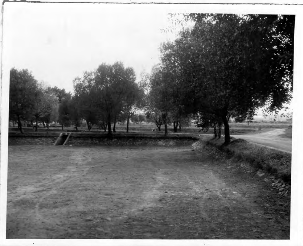
Figure 2. Drained muskellunge pond at Spooner Hatchery, Wisconsin. Note the rip-rapped sides and the cleanness of the hard bottom. This pond is a very good producer of muskellunge fingerlings. Photo taken August 26, 1952.
