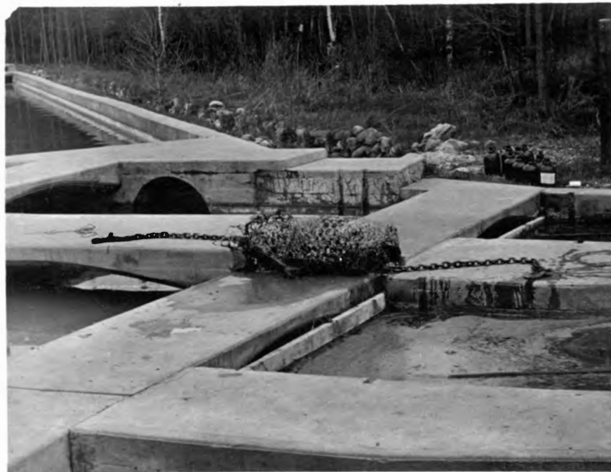
Figure 6. Roll of chicken wire and heavy chain for agitation of bottom of raceways.
