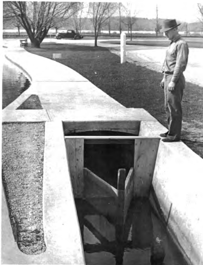
Figure 10. Screen at end of waste ditch. The top was covered after the photo was taken to prevent fish from jumping over the screen.
