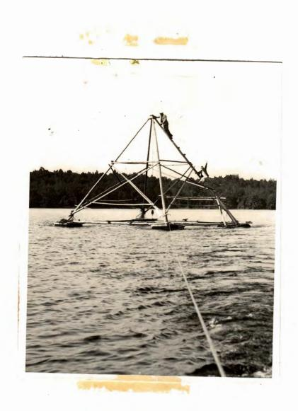
Fig. 1. Hoist used in lifting brush shelters. The device is being towed to the site of a shelter.
